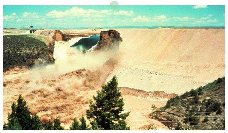
The 1976 Teton Dam failure in Idaho shows the high velocities in the resulting flood. This occurred on a sunny day, catching many downstream occupants by surprise. Photo by Eunice Olson, courtesy of A. G. Sylvester.
