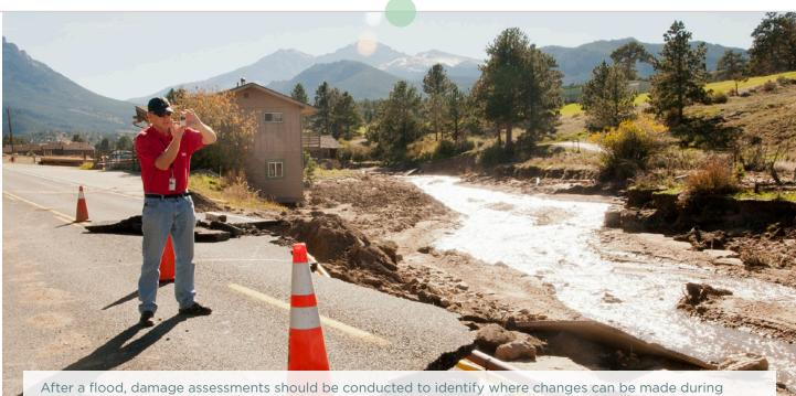
After a flood, damage assessments should be conducted to identify where changes can be made during repairs and reconstruction. Damage assessments are vital for a post-disaster plan, such as the ones discussed in Section 3, Tool 3, Estes Park, CO. Photo by Patsy Lynch/FEMA.
