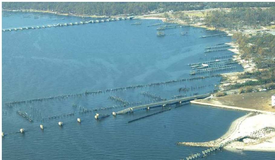
Bay St. Louis bridge and highway destroyed following Hurricane Katrina
