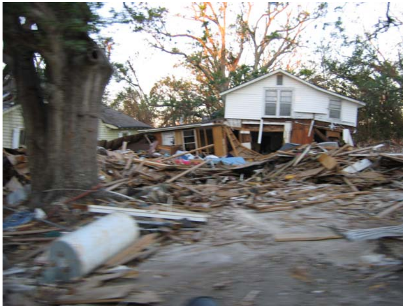
Damaged house, Biloxi
