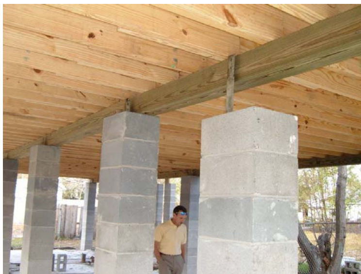
Hurricane bracing, MS
