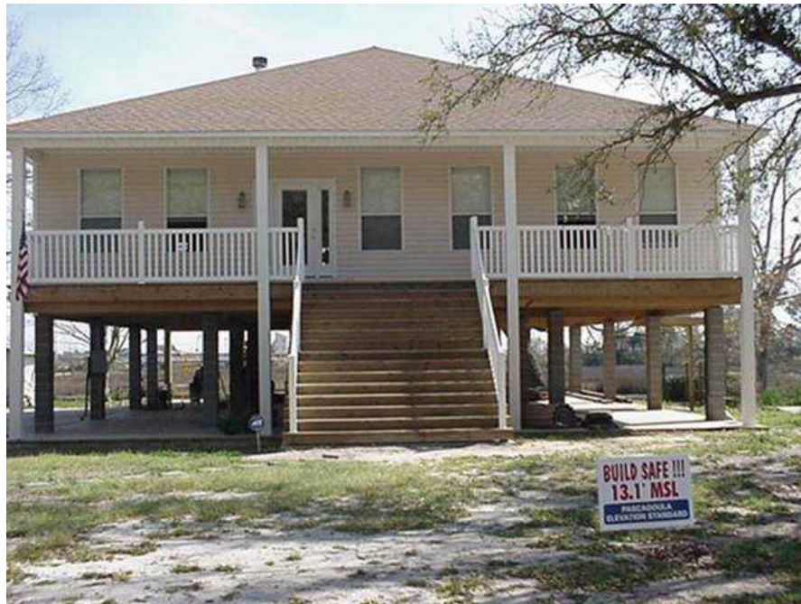
Pre-Katrina elevation helped to save this house
