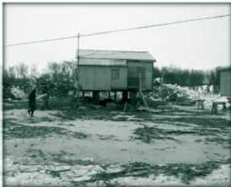
Relocating a house (Alaska)
