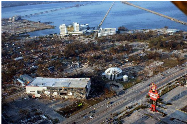
Post Katrina damage, Biloxi, MS
