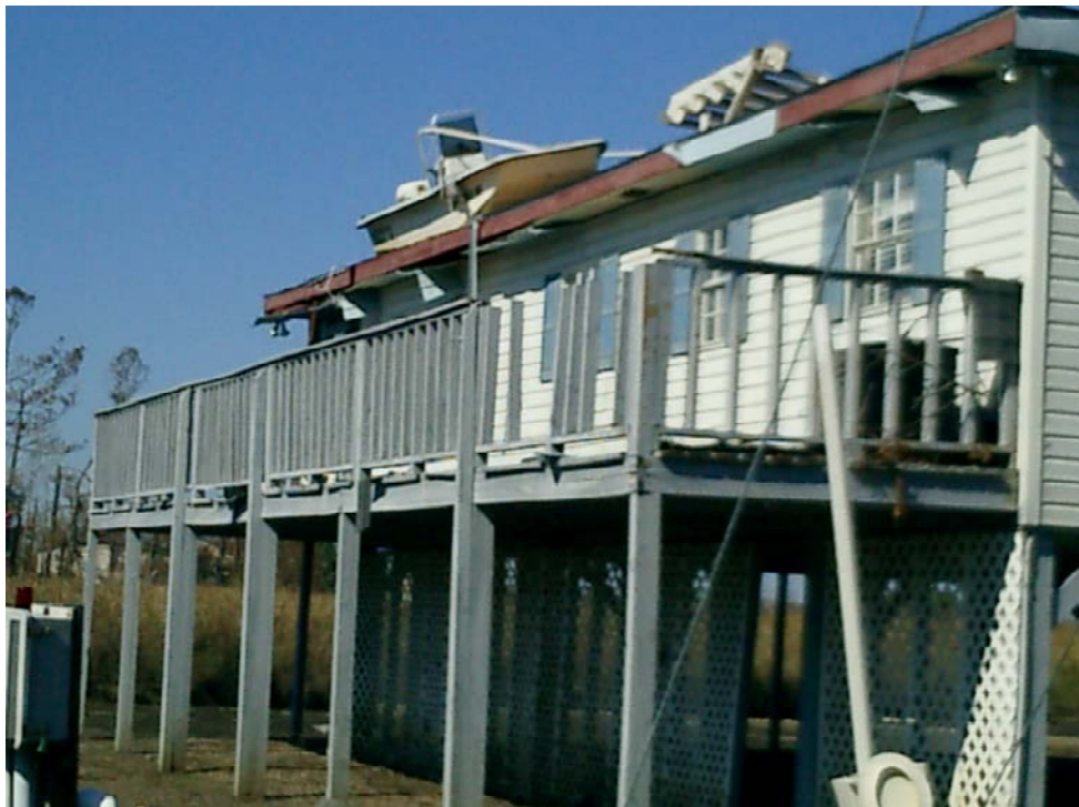
This structure not elevated enough to avoid having a boat being left on its roof by Katrina
