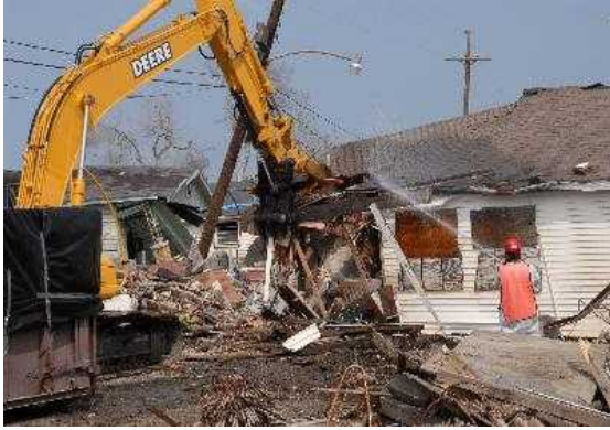
Demolishing a house
