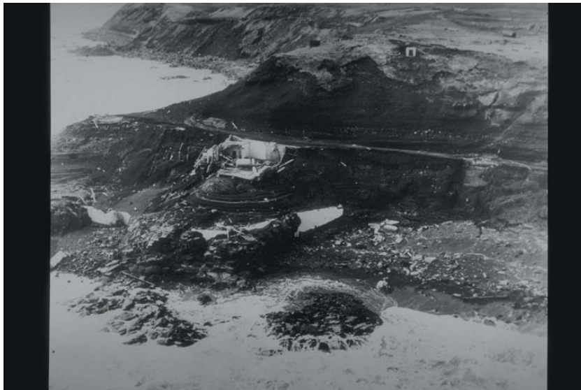
Lighthouse destroyed in tsunami
