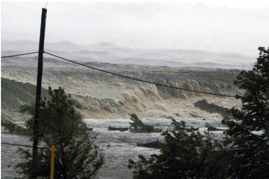
Katrina coastal surge topping levee
