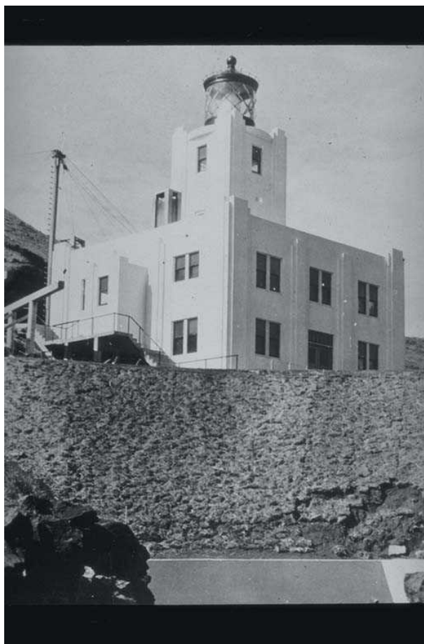
Lighthouse before tsunami
