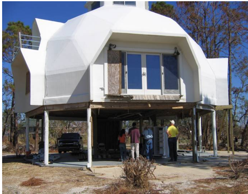
Geodesic dome style to resist wind forces
