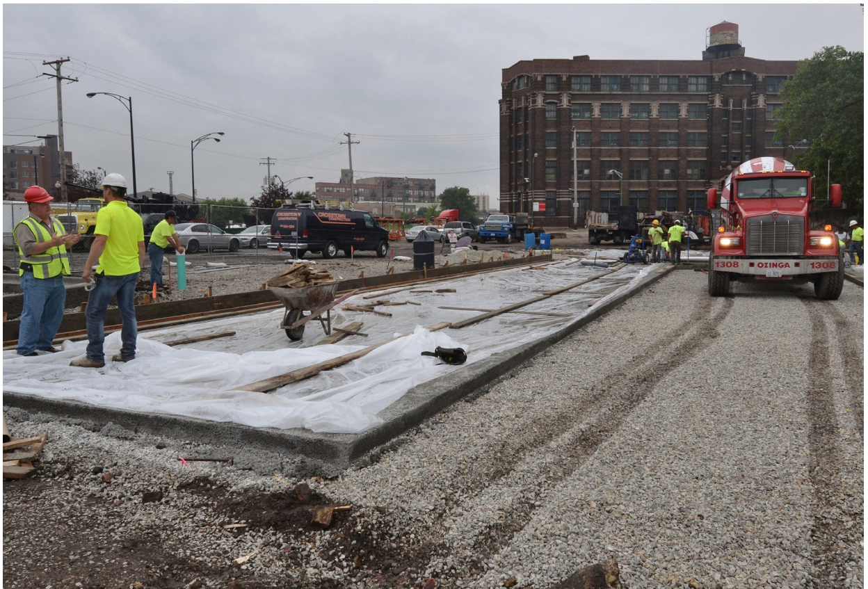
Installing porous paving, a RainReady solution, in Chicago, IL
