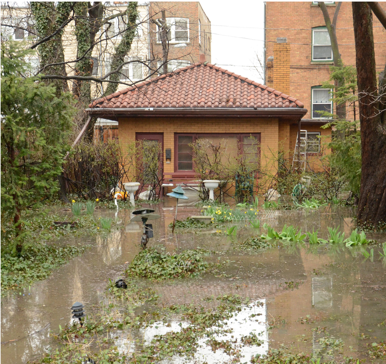
Backyard flooding in Chicago
