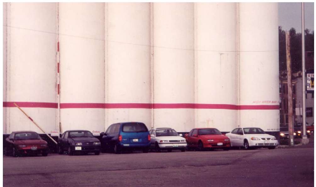
The red line on the grain elevator in Alton, IL, shows the height of the 1993 Mississippi River flood. The lower, black, line marks the 1973 flood. Photo credits: French Wetmore.
