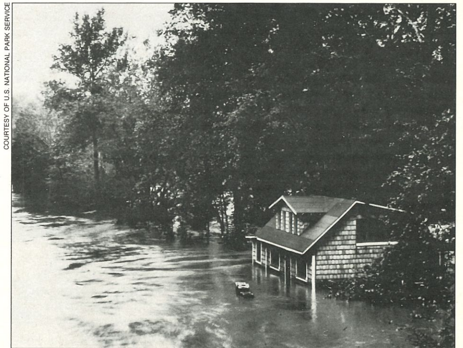
The costs of rebuilding after a flood today are much higher than those of historical floods, such as this one, which closed the Chesapeake & Ohio Canal in 1924.
