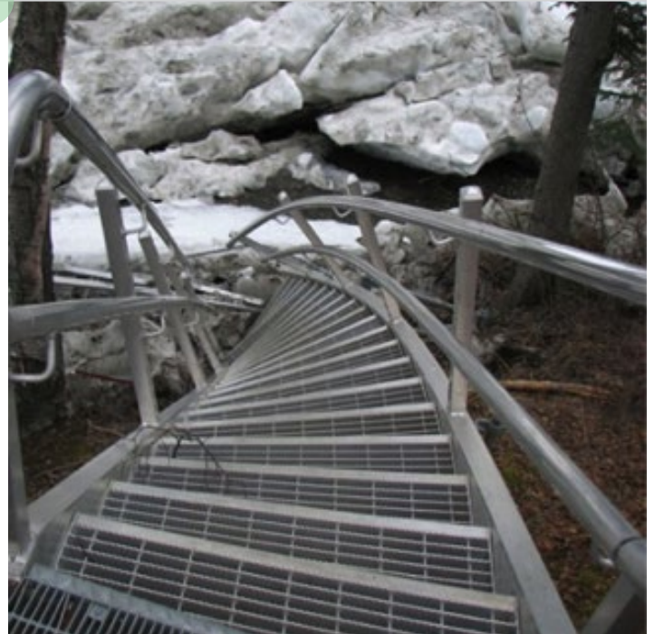
Kenai River Center stairway to the Kenai River twisted by the force of the 2007 ice jam flood event. Photo courtesy of the Kenai River Center
