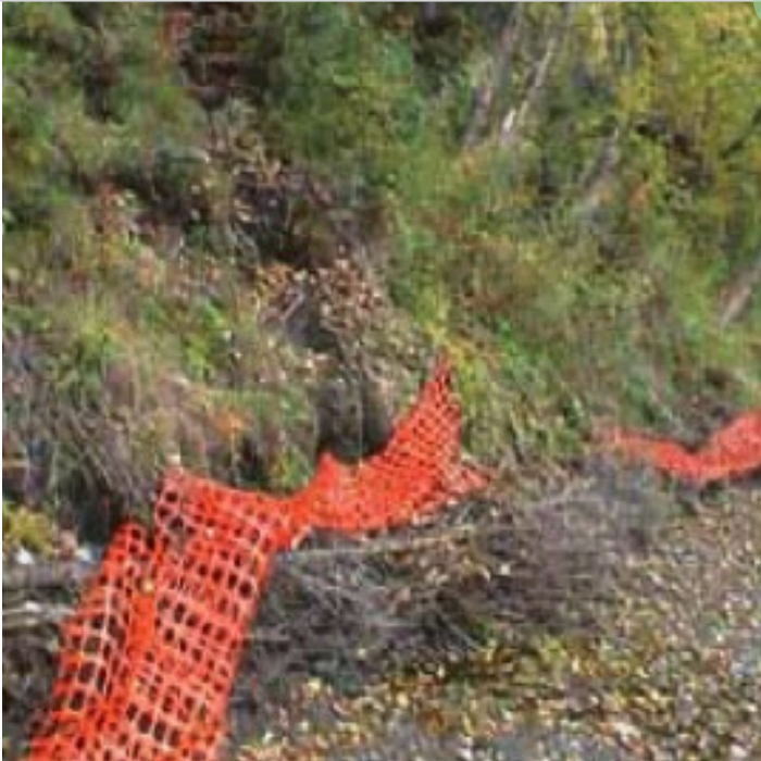
Old restoration effort and eroded hill
