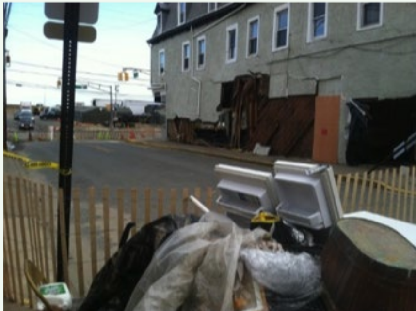
Hurricane Sandy aftermath (Photo credit: John Miller, PE, CFM, CSM, Associate Water Resources Engineer; Princeton Hydro, LLC)
