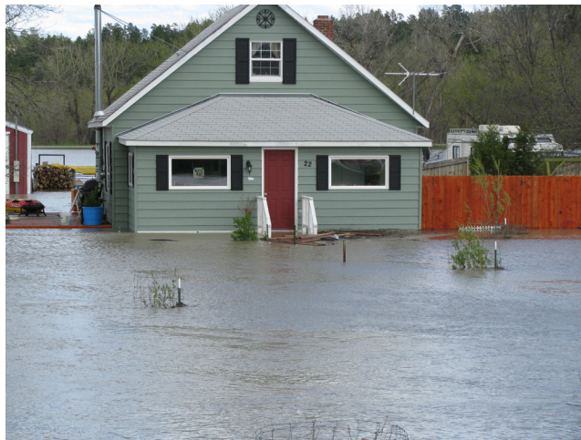
Figure 6.1. Flood waters from the Musselshell River inundate this home in the city of Roundup, Montana, during the record-setting 2011 flood event (Musselshell County, Montana)
