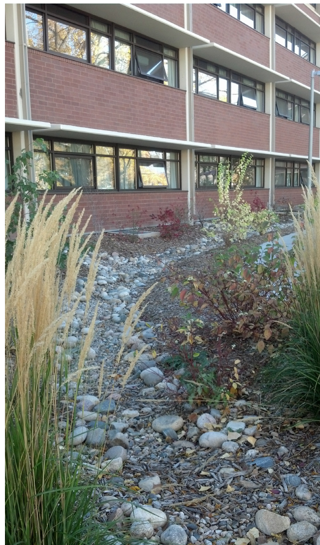
Figure 5.9. Bioswales in a parking lot (above), along a pedestrian path (below), and in front of a building on the campus of Colorado State University (right) (Chad Bergjinnis)
