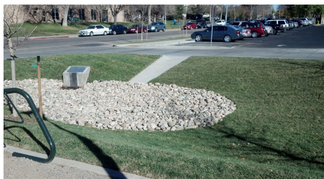
Figure 5.9. Bioswales in a parking lot (above), along a pedestrian path (below), and in front of a building on the campus of Colorado State University (right) (Chad Bergjinnis)
