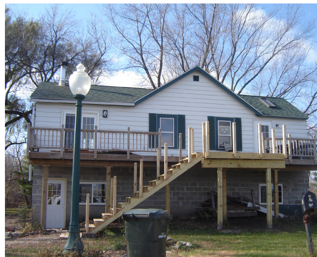
Figure 2.4. A home elevation project in progress, November 2008 (James C. Schwab)
