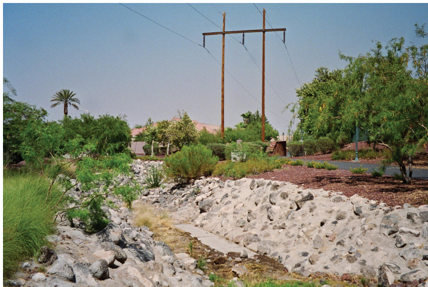
Figure 2.6. Stormwater management infrastructure in Henderson, Nevada (Carolyn Torma)
