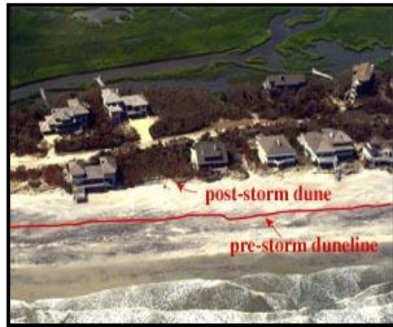
After Hurricane Fran, September 1996.
