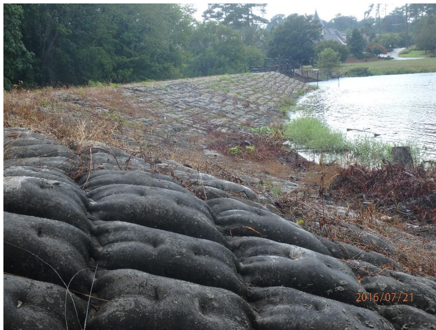
Figure 24: Concrete Armoring at Forest Lake Dam (Source: FEMA)
